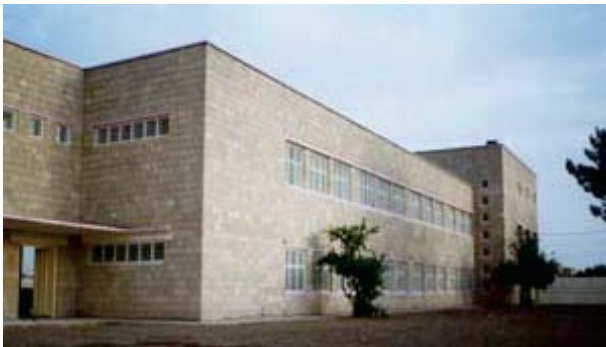
Shorish Preparatory, rehabilitated by UNESCO
