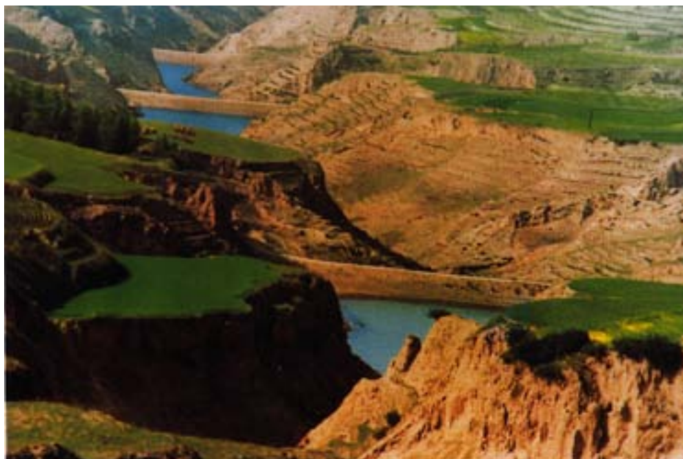
Figure 3 Key Dams for Gully Erosion Control
