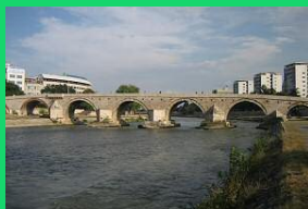
The Stone Bridge, Skopje © OLDSKOPJE
