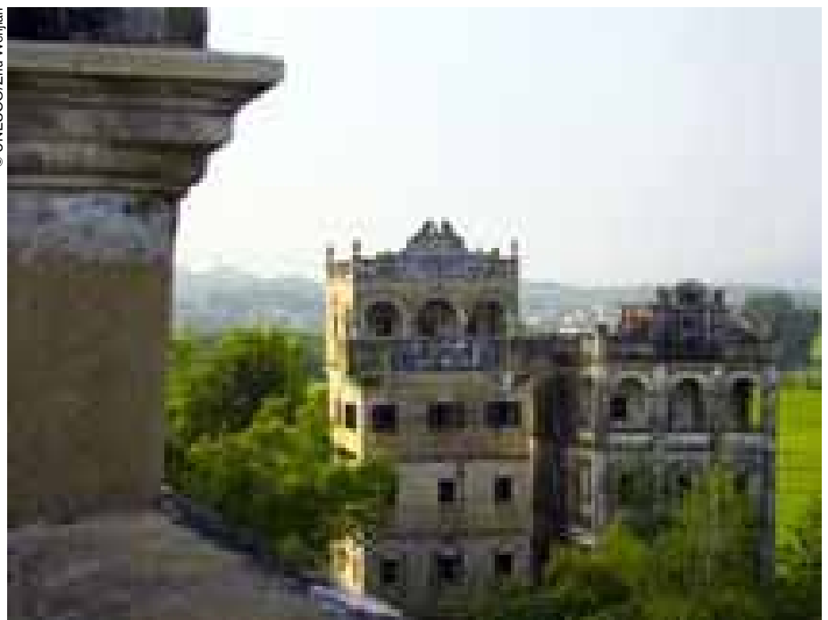
An Lu, fortified towers in Zili village (Kaiping).
