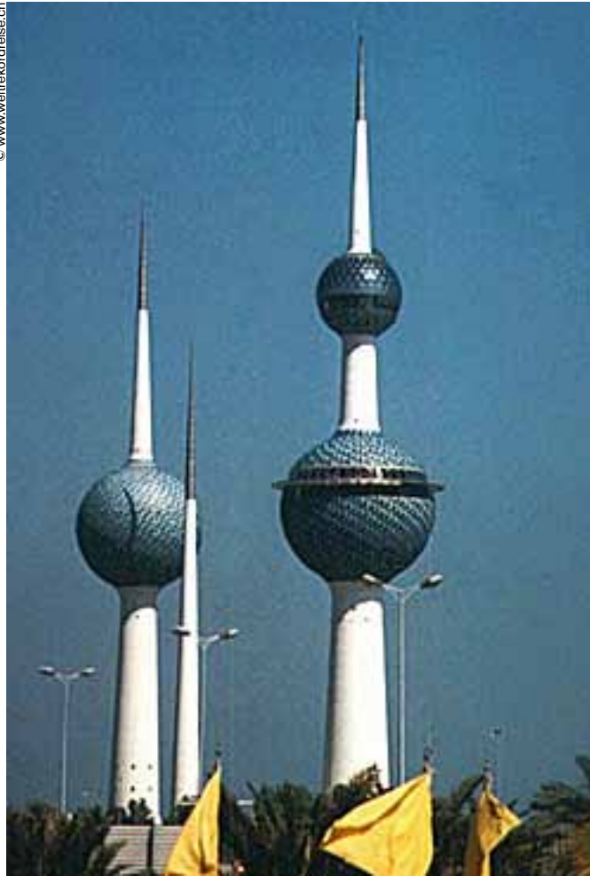
Water towers in Koweit.
