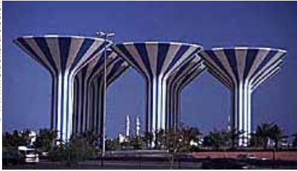
Stripped water towers in the Gulf region providing precious water supply.
