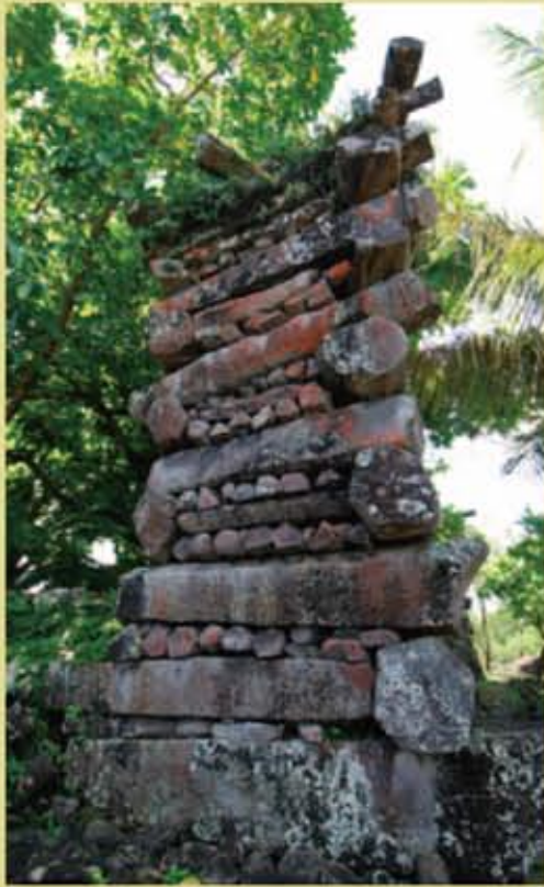
Entrance in the outer wall of Nandauwas. The wall is built of prismatic basalt piled in alternating header-stretcher courses, and rises to a height of approx. 8 m.
