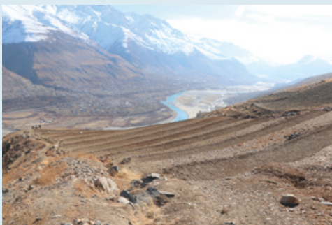
Terraces constructed to stabilize slopes and limit soil erosion
