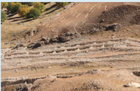
Check-dams, soil bunds and tree plantations to help stabilize slopes
