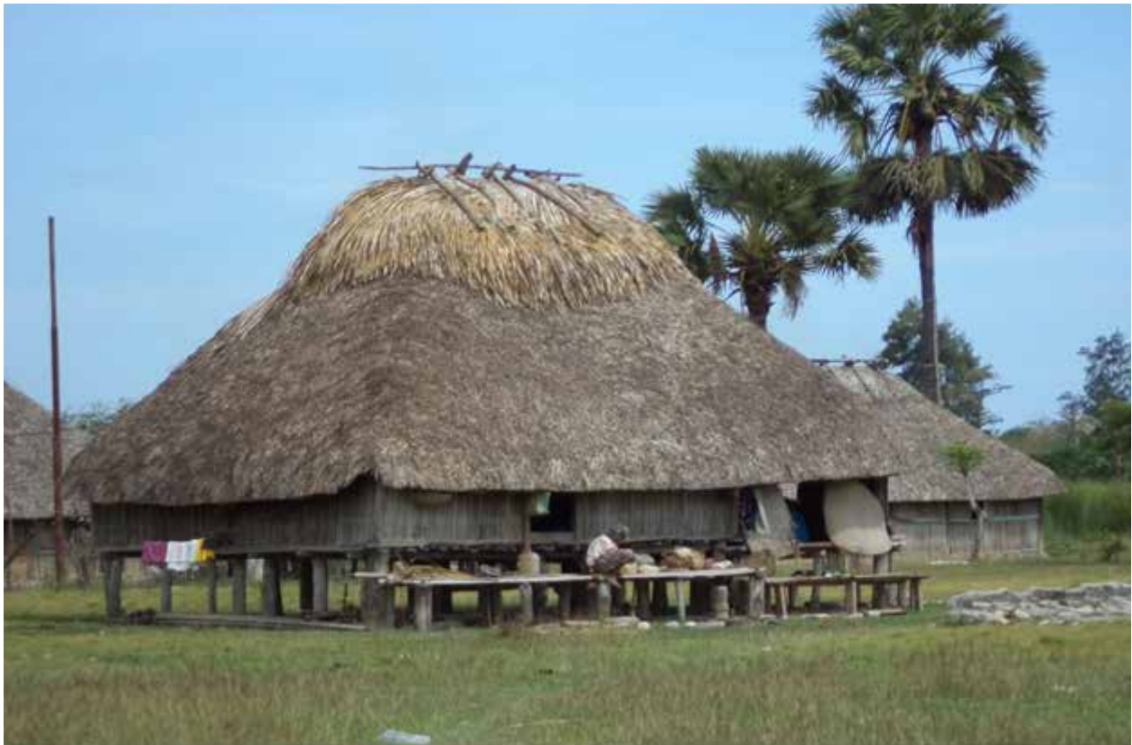
Figure 2.3.2: Traditional house in Raimea Village, Covalima, Timor-Leste, with Ai Tatan to clamp the roof from storms and strong winds, and Lenik to prevent strong winds from entering the house.
