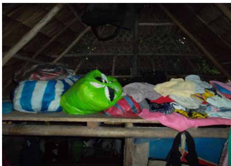
Figure 3.2: Tinabaw, a loft-like part of a house that serves as a place to keep occupants and their belongings safe in times of floods and typhoons (practised in Perez, Alabat Island, the Philippines)
