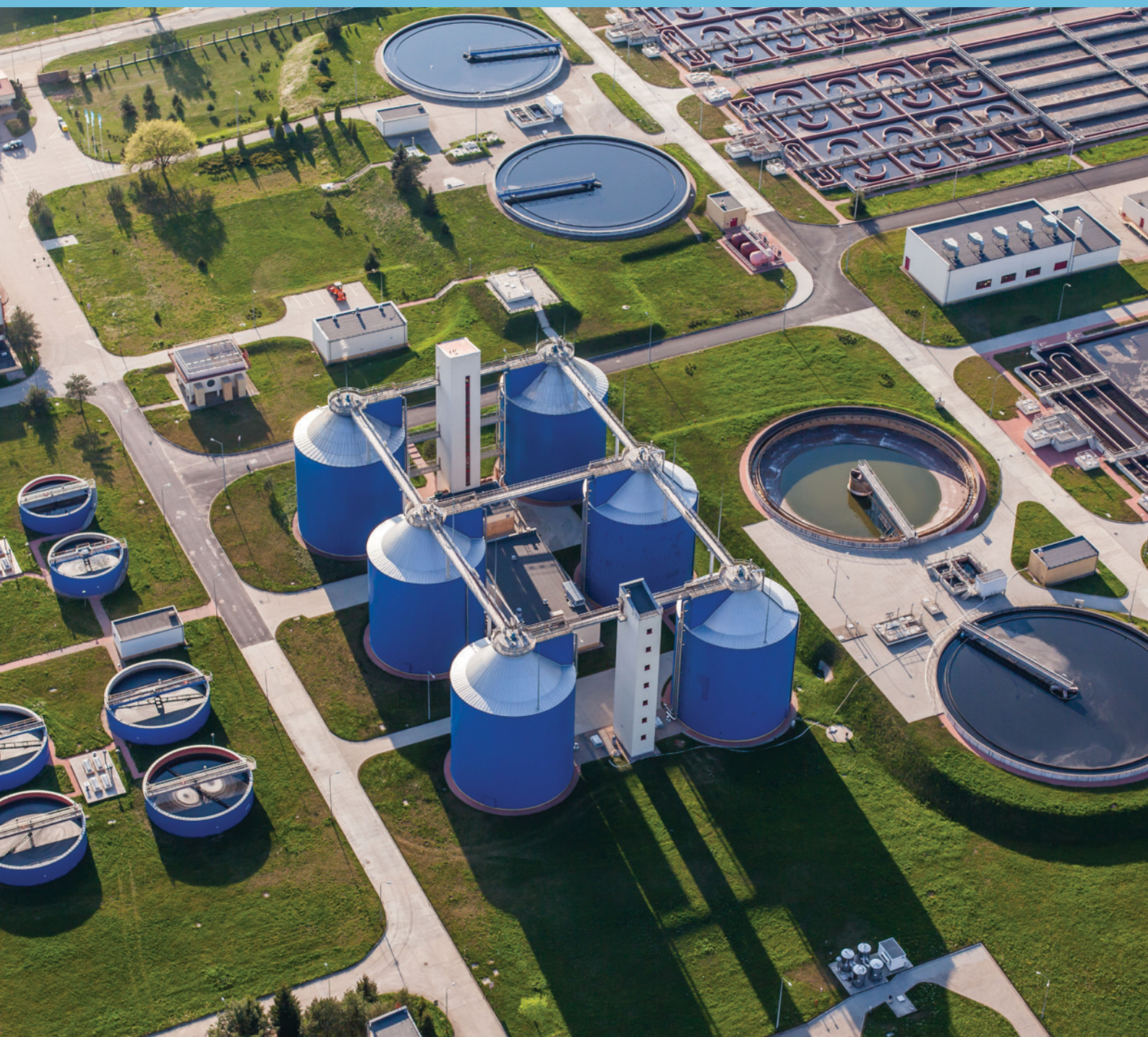
Aerial view of sewage plant treatment in Wrocław (Poland).
