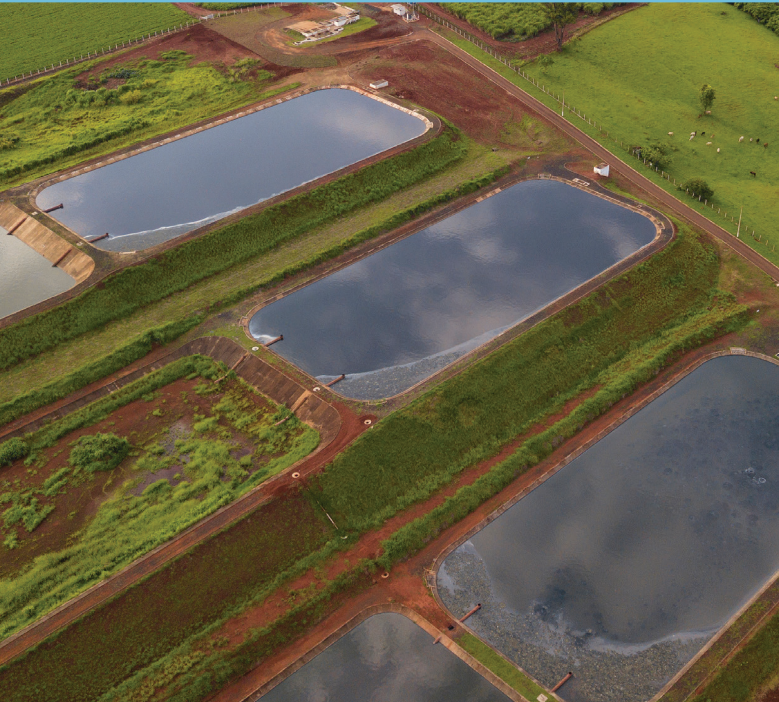
Aerial view of a sewage treatment facility.
