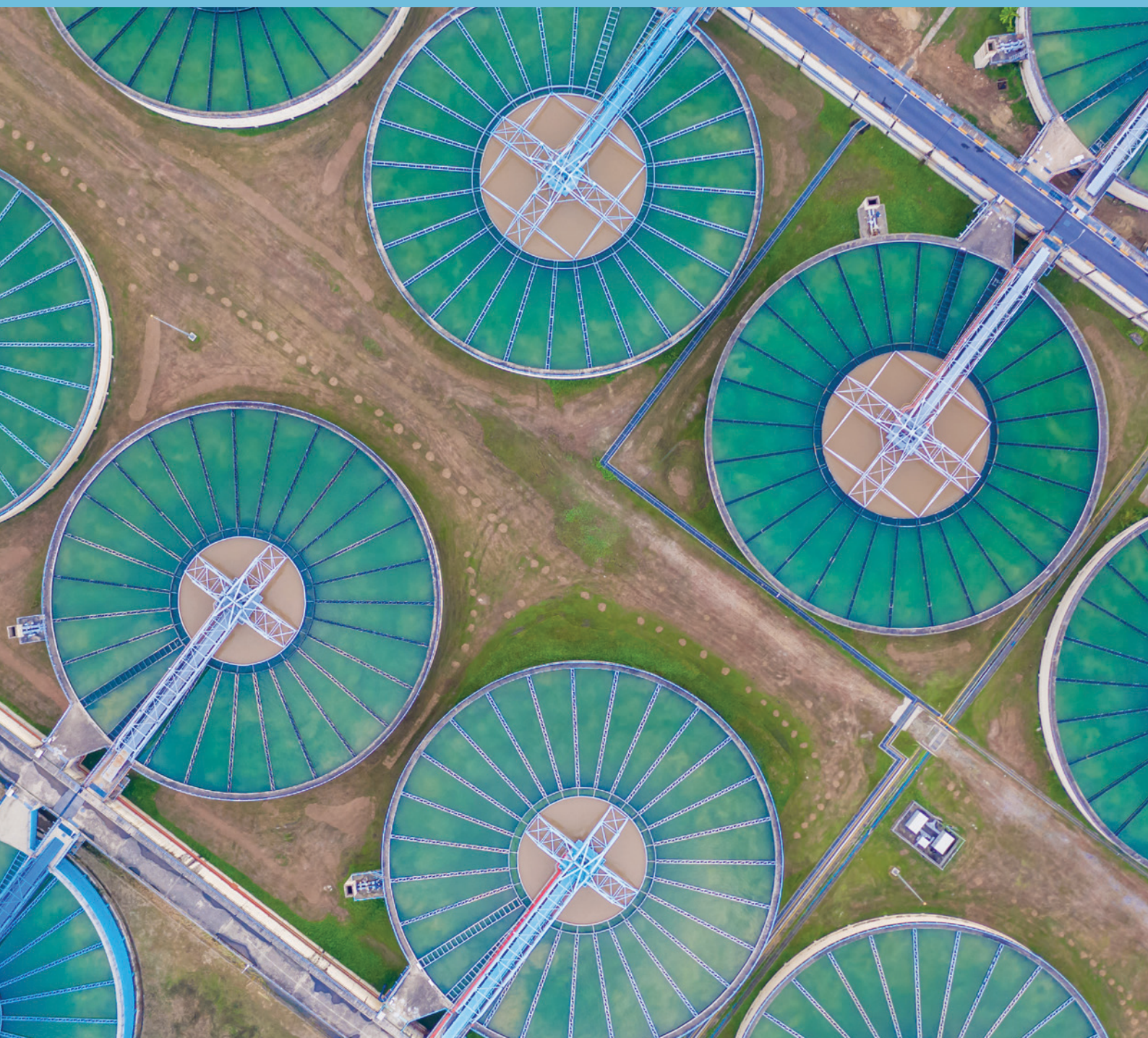
Aerial view of a water treatment plant.
