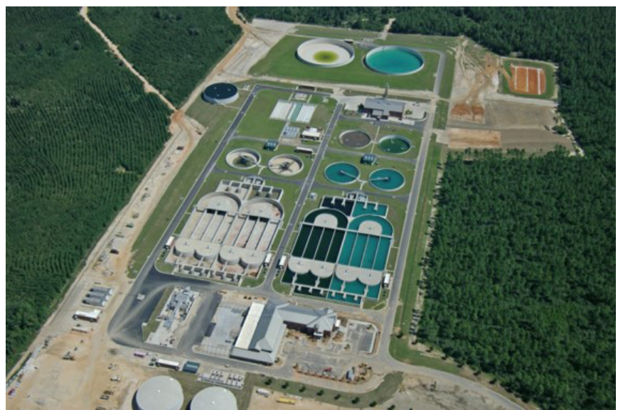
The wastewater treatment plant in Escambia County, Florida (USA), destroyed by Hurricane Ivan, and replaced and relocated away from the coastal plain and built to be more resilient. The plant now reuses 100% of its water.
