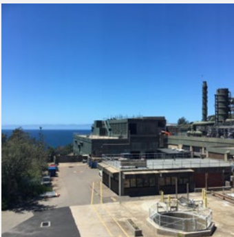
Biogas from treated sewage used to generate electricity at North Head Wastewater Treatment Plant, Sydney, Australia. © Marlene Kanga
