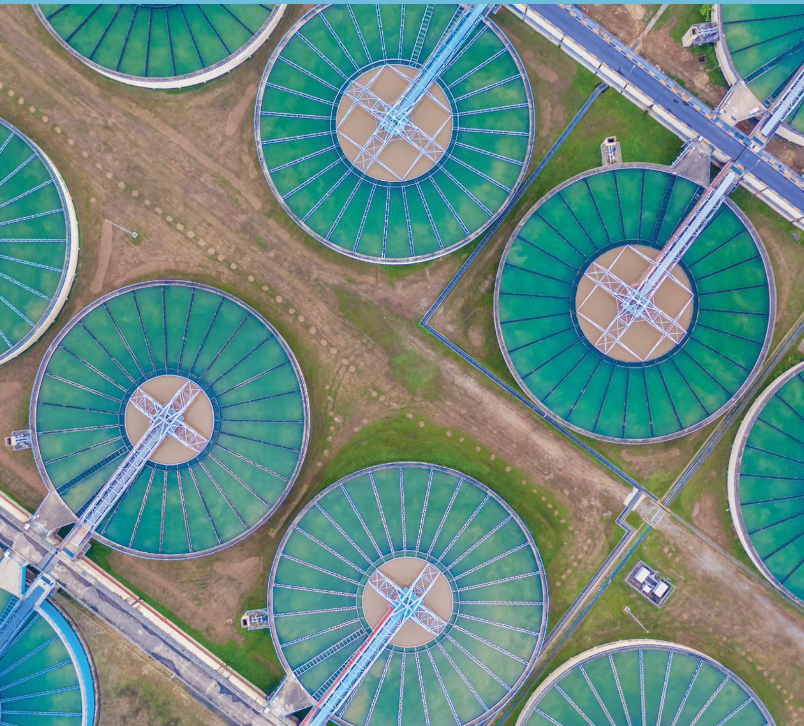
Aerial view of a water treatment plant.
