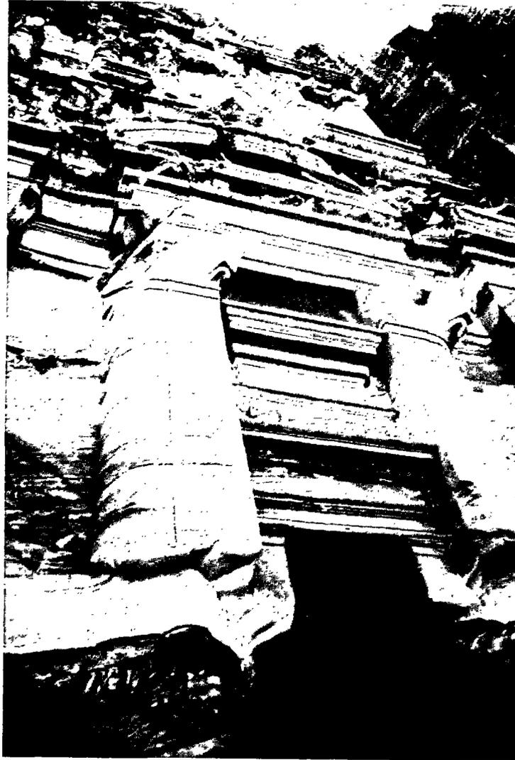
Total destruction of the architectural details at the base of the Palace Tomb due to the capillary circulation of water through the rock. Erosion 'per ascensum'.
