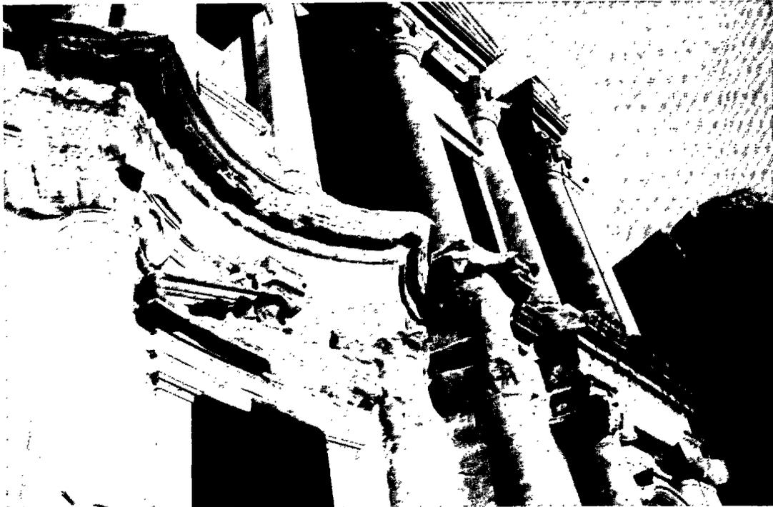
Al Deir. Scarcity of ground cover due to trampling and grazing increases the problem of erosion. Destruction of architectural detail caused by rainwater runoff where the cornice has been worn away.
