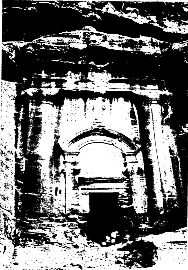
The 'Renaissance Tomb', in Wadi Farasa. Note the formation of a Tafoni below the urn, the vertical traces of run-off on the facade directly below the destroyed portions of the cornice, and the weathering at the base of the monument.
