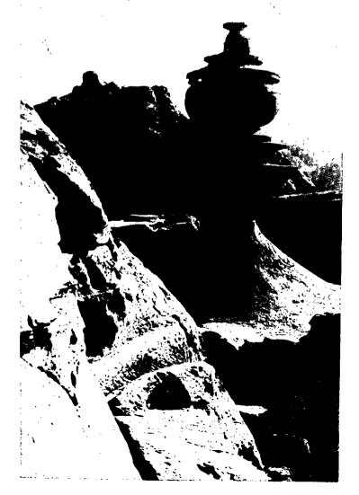
Al Deir. Rainwater channels and gutters also served to protect the stone façades against erosion due to runoff Lane
