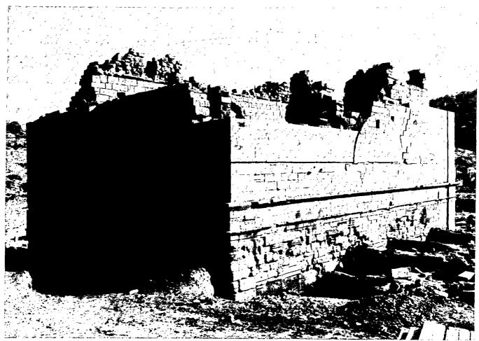
Qasr al Bint. South-west corner before and after restoration. Note loose stones displaced by an earthquake in antiquity. Unprotected excavation trenches left open at the base of walls may put the foundations at risk from rain.
