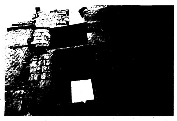
Reconstructed south-east corner showing extant section of cornice and freize leaning out of plumb. Note ugly and inappropriate use of exposed concrete to strengthen staircase.
