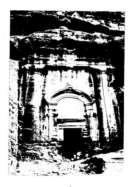
The 'Renaissance Tomb', in Wadi Farasa. Note the formation of a Tafoni below the urnm the vertical traces of run-off on the facade directly below the destroyed portions of the cornice, and the weathering at the base of the monument.
