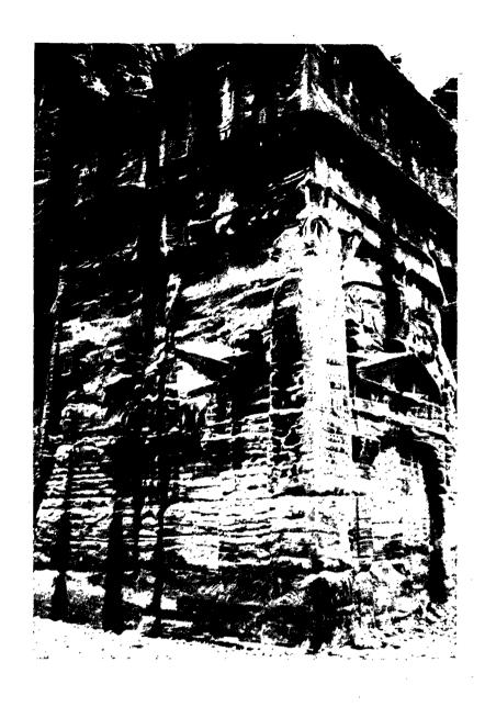
Obliteration by erosion of the architectural details of a rock-carved monument (Brünnow Tomb). Note the enlargement of the diaclase, the alveoles exploiting the stratification, and the start of the formation of tafoni below the cornice.
