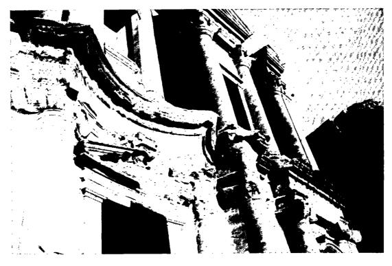
Al Deir. Scarcity of ground cover due to trampling and grazing increases the problem of erosion. Destruction of architectural detail caused by rainwater runoff where the cornice has been worn away. Lane
