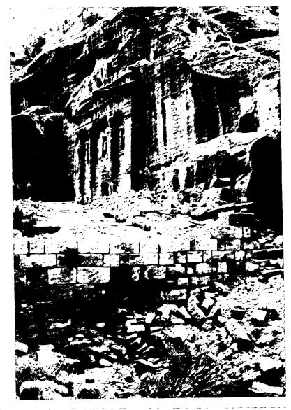
The gullying of a terrace in Wadi Ghurab is the result of the recent collapse of a retaining wall.
