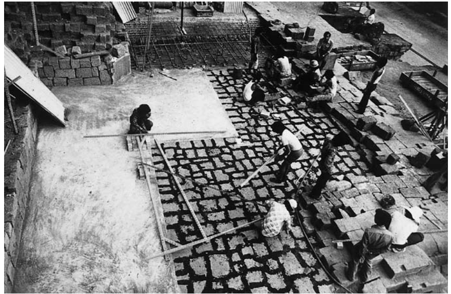
Photo 6.2.4.1 Rebuilding scheme North/South Source: Borobudur Restoration Project
