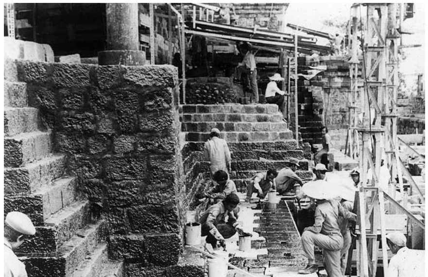
Photo 6.2.4.2 Rebuilding scheme East/West Source: Borobudur Restoration Project
