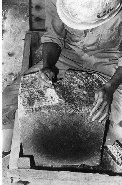
Photo 6.2.2.6 Elimination of rhizomes of mosses in the pores of the stones using a fine needle
